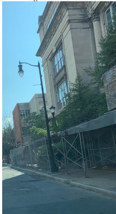
Here is the same school building in its patented school board ugly filthy regalia Picture by Kathleen Kelly
