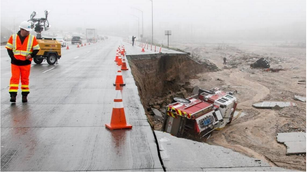
A San Bernardino County firetruck plunged off Interstate 15, when a lane and shoulder caved in due to heavy rains in the Cajon Pass on Feb. 18. IRFAN KHAN LOS ANGELES TIMES
