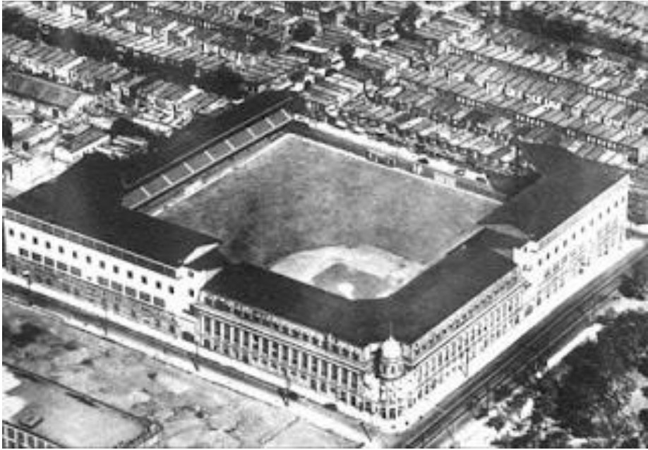
1909 Shibe Park Opened. It became Connie Mack Stadium, Philadelphia
