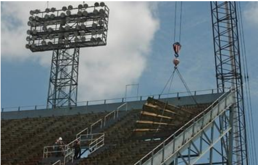
Because of structural problems that were too costly to repair, the Legion Field upper deck was torn down in 2005. (Joe Songer/jsonger@al.com)
