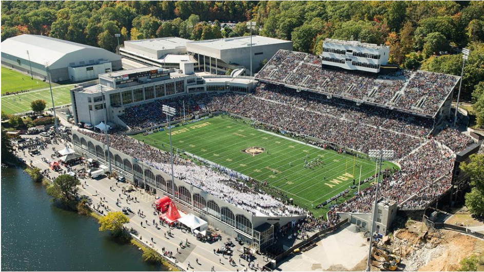
Blaik Field at Michie Stadium West Point NY
