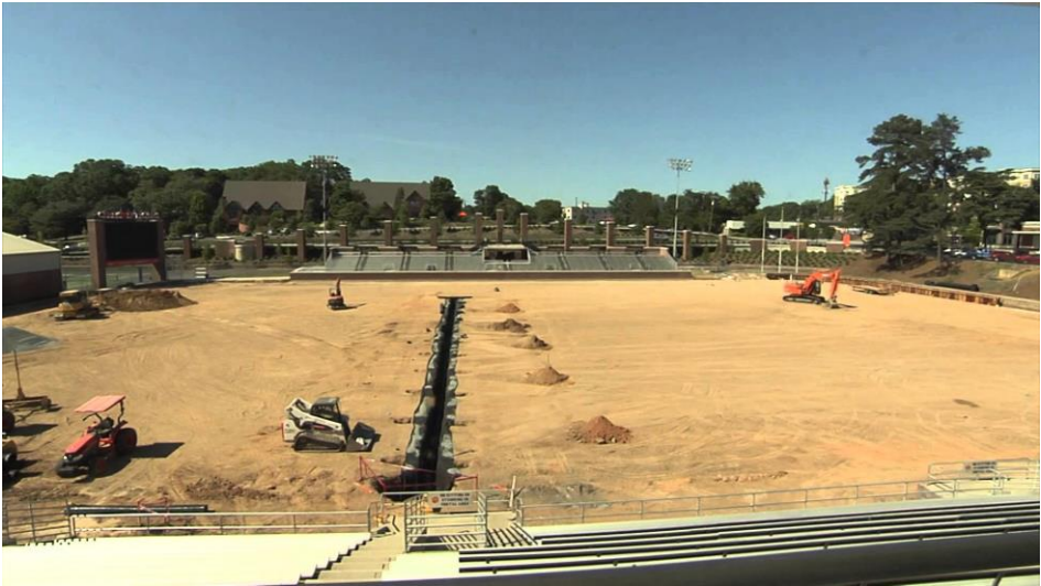
Riggs Field 2015 Construction
