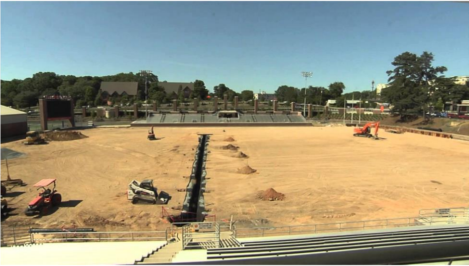
Riggs Field 2015 Construction
