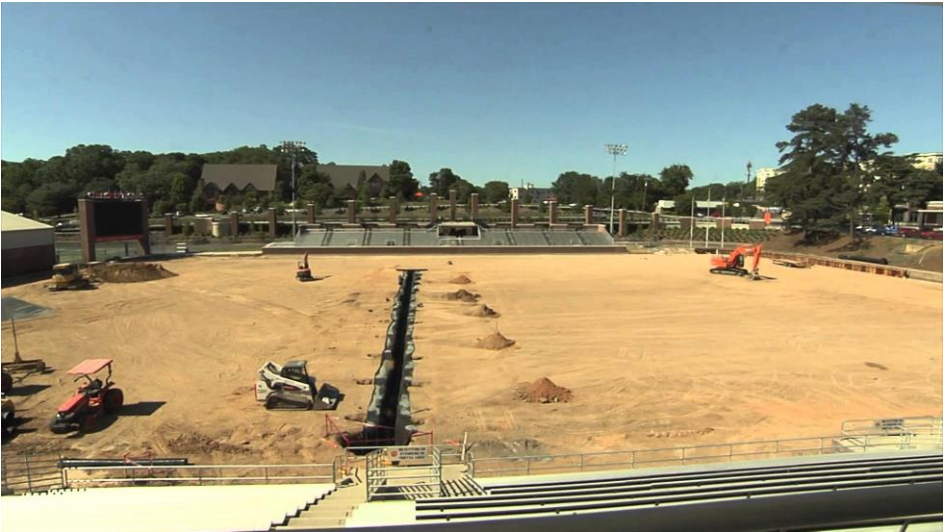
Riggs Field 2015 Construction
