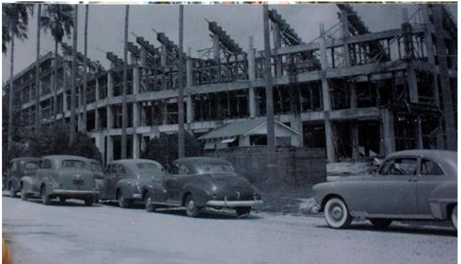
Construction of the west stands, August 1950.
