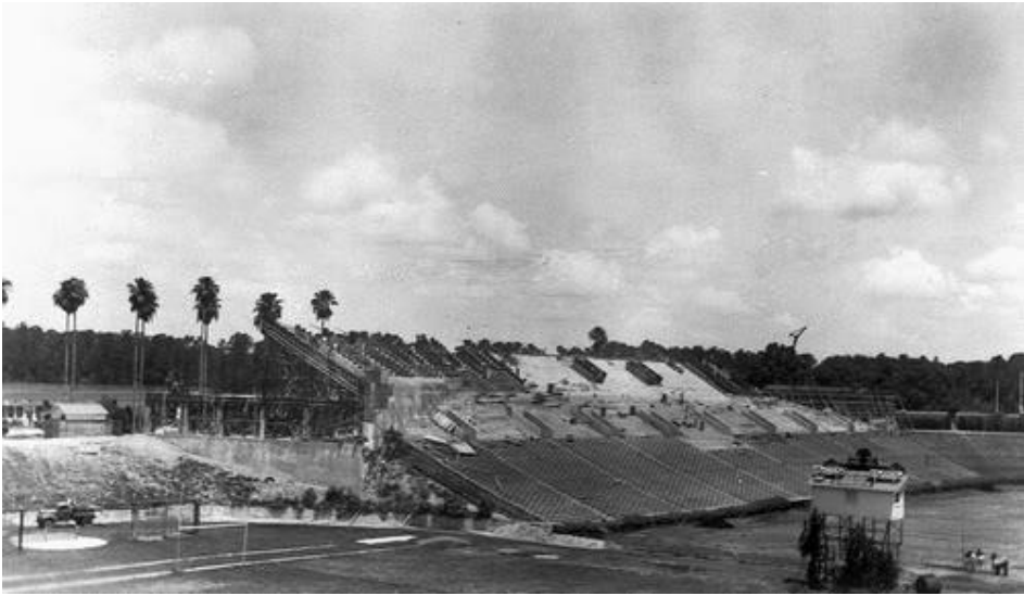
Construction Continues Florida Field in 1930
