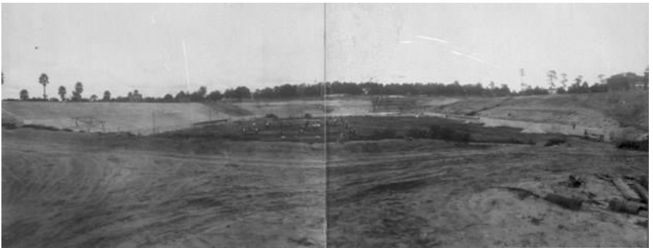
Construction Begins on Florida Field in 1930
