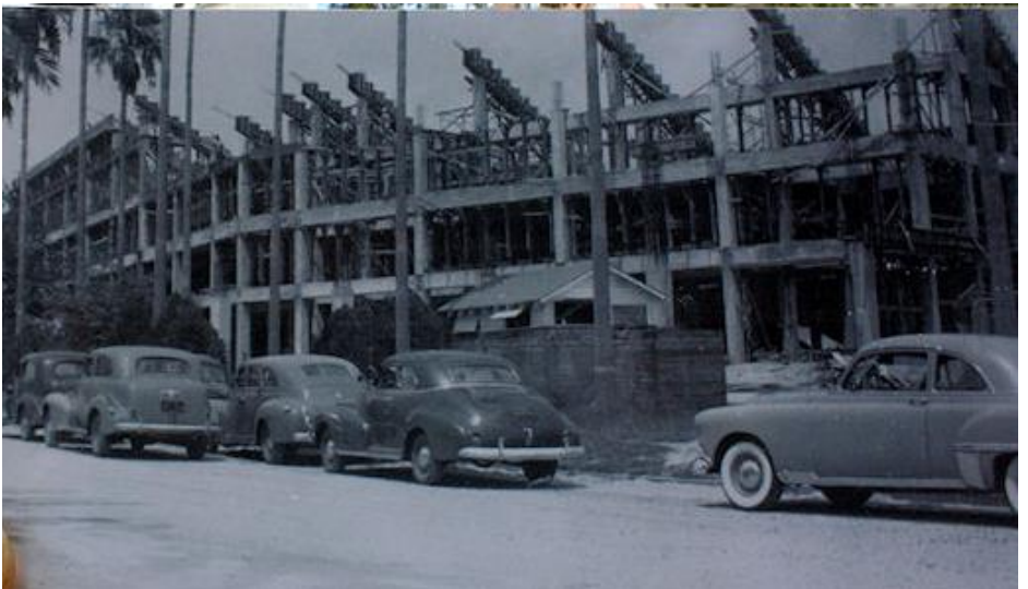
Construction of the west stands, August 1950.
