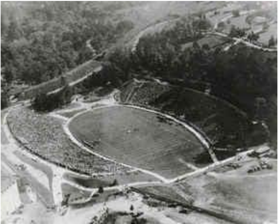
Early Sanford Stadium
