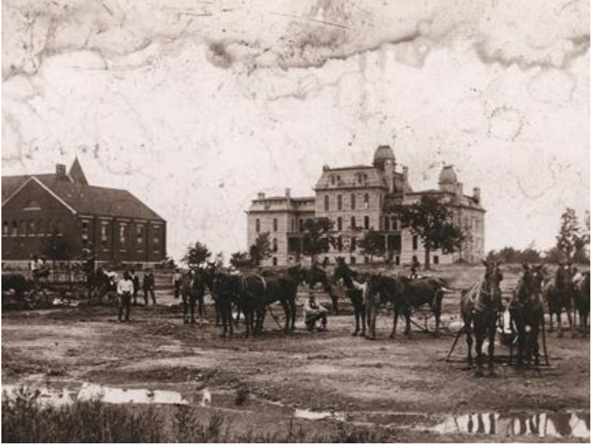
The Oval Field being built with horse-power
