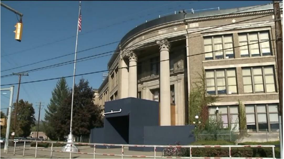
Front Entrance particle board and PVC mirror the same look at the side entrance of Meyers
