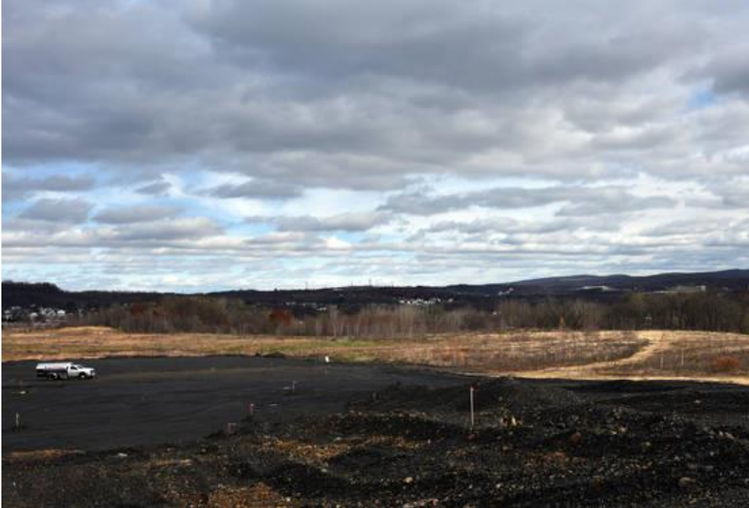
The truck in the distance sits roughly to the right of what is to be the main entrance of Wilkes-Barre Area’s new consolidated high school. - Aimee Dilger | Times Leader
