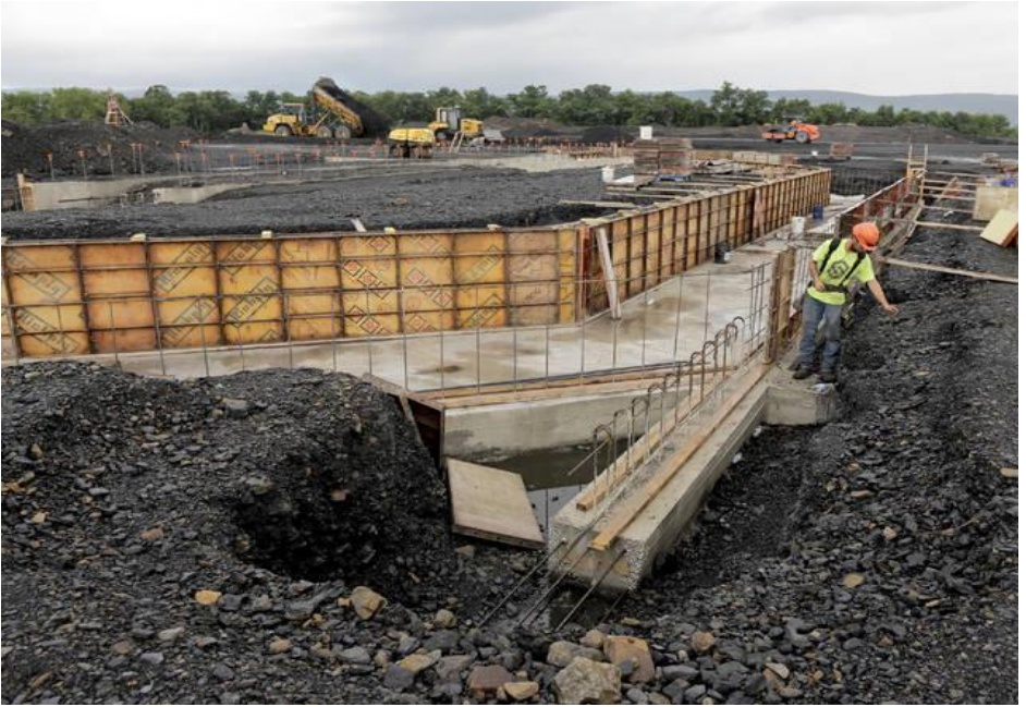
The front of the auditorium stage is outlined as workers continue construction of Wilkes-Barre Area's new consolidate high school. Bill Tarutis | For Times Leader
