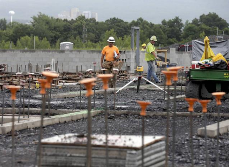
Pictures Work proceeds among foundation footers with reinforced bar jutting up to support concrete masonry unit walls — like those partially completed in the background — at the construction site of WB Area’s consolidated high school. Bill Tarutis | For Times Leader
