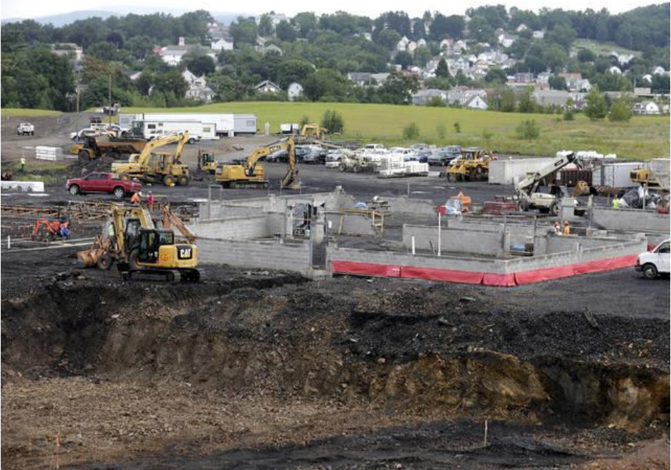
Construction continues on the swimming pool, front, in the athletic wing of the new Wilkes-Barre Area High School in Plains Township . Bill Tarutis | For Times Leader
