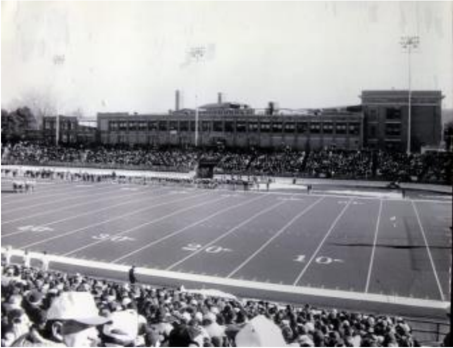
Meyers with bleachers hugging school and artificial turf
