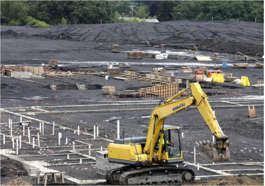
Workers have begun building concrete masonry unit walls at the site of the Wilkes-Barre Area consolidated high school. Foundation work is well underway at the construction site of Wilkes-Barre Area's consolidated high school. . Bill Tarutis | For Times Leader
