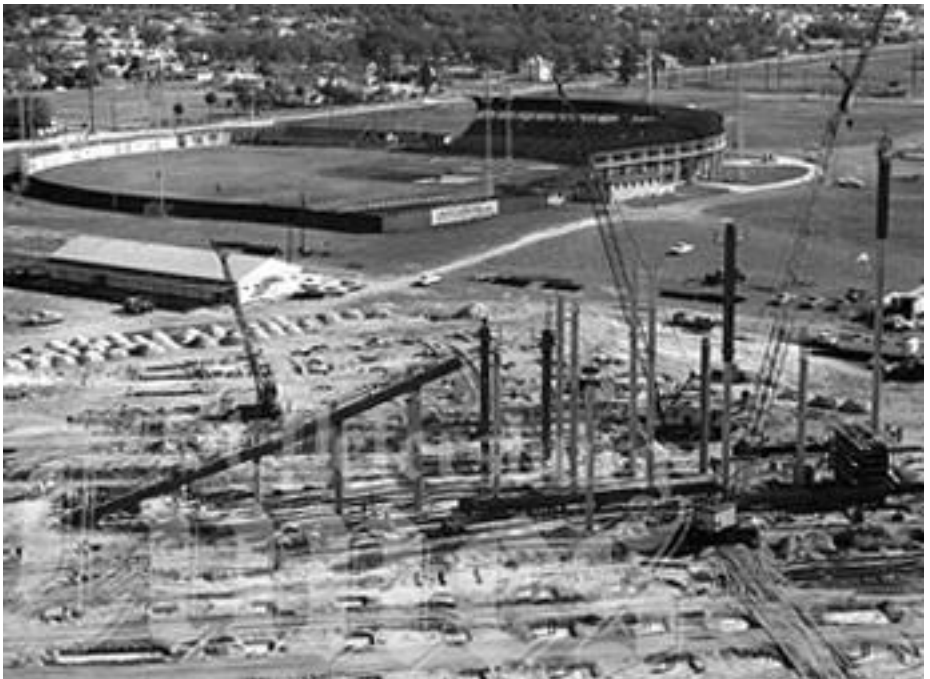
Tampa Stadium construction, Jan. 1967
