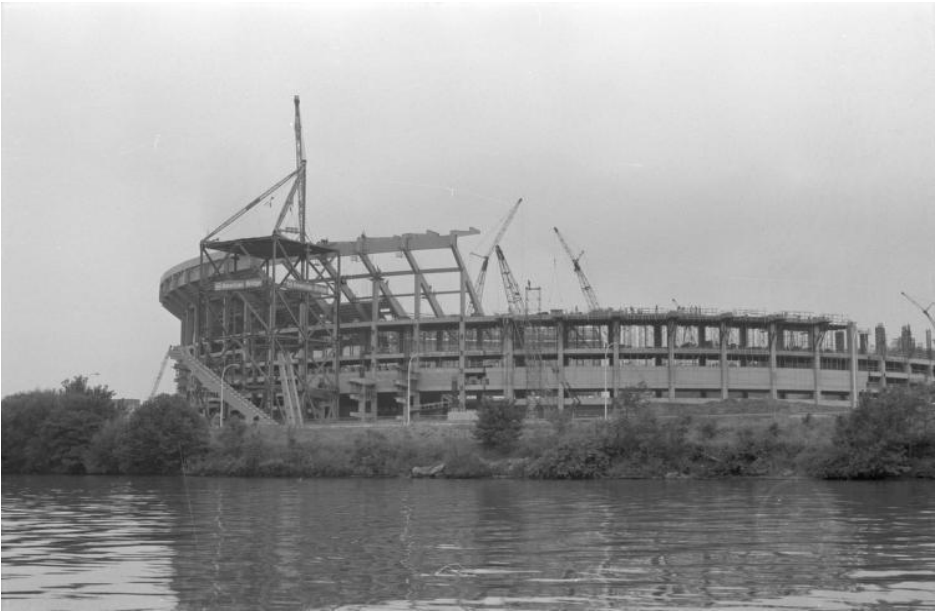
The new stadium rises from the rubble in 1969.
