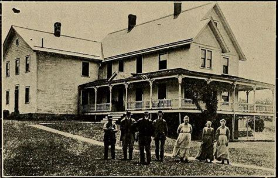
Classic Poor House
