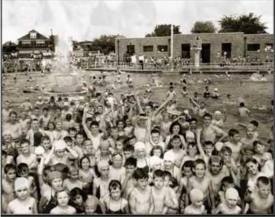
Miner Park Swimming Pool South Wilkes-Barre See Fountain in Middle
