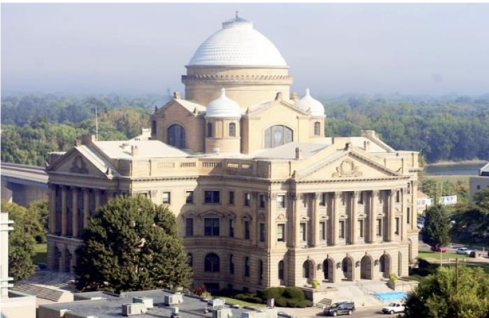
Luzerne County Courthouse in WB -- a monument to good planning 1909
