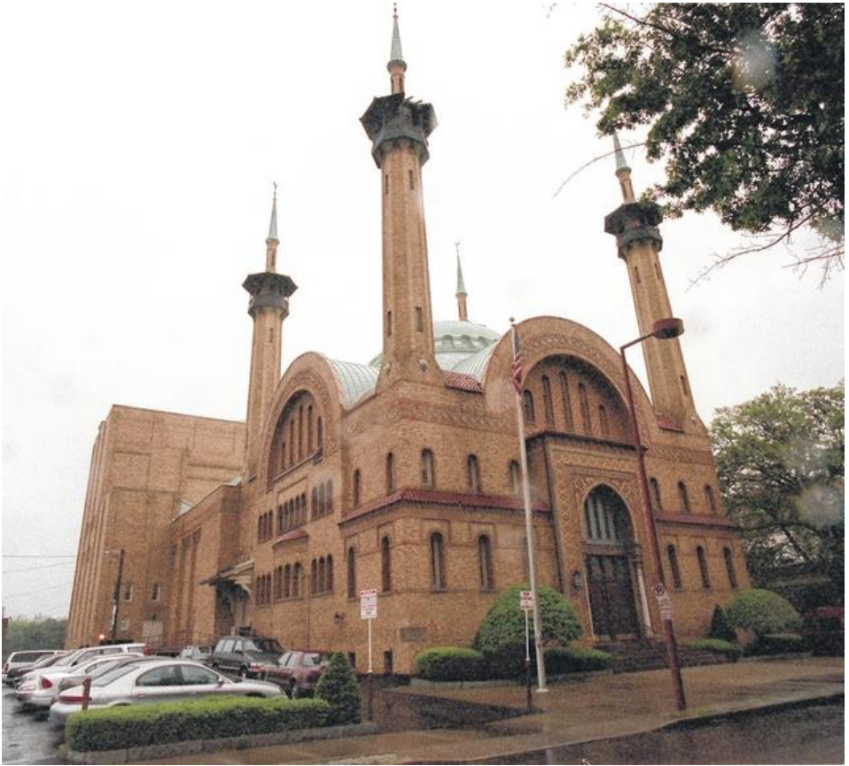
The magnificent Irem Temple—repairs are progressing
