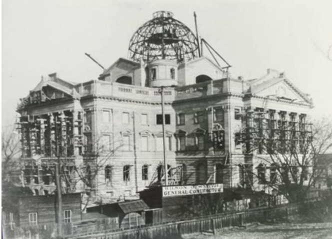
Luzerne County Courthouse circa 1908 River Street, under construction
