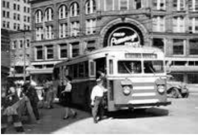
Pomeroy's in the 1950's before the Façade "Lift"
