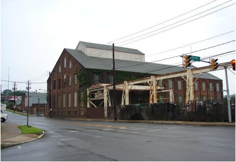
Site of the Vulcan Iron Works Where Huge Locomotives Were Once Built
