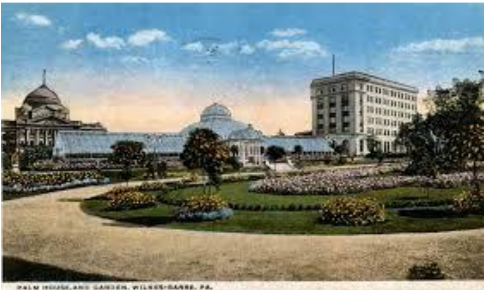
In the background, the Coal Company Building became King's College-- a great perspective.
