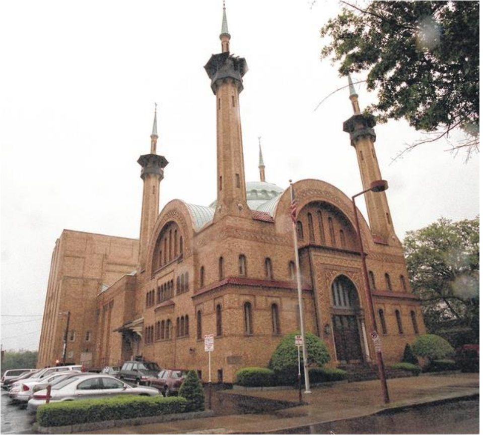
The magnificent Irem Temple—repairs are progressing
