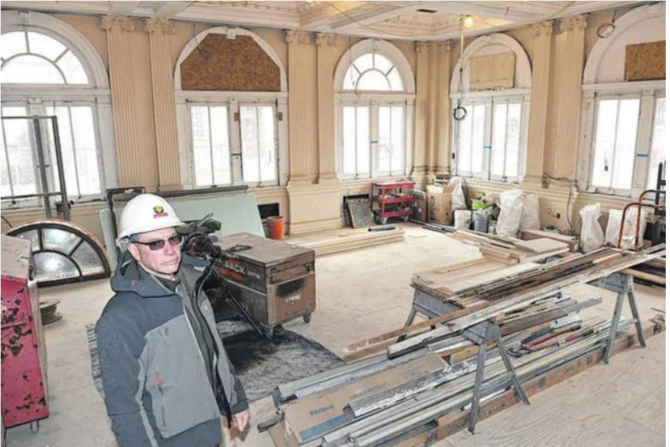
Springbrook Water / King's project in process
