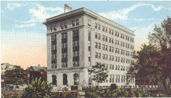
Lehigh Valley Coal Company Building pre-King's 1916 Notice the later addition of Christ the King had not been completed.
