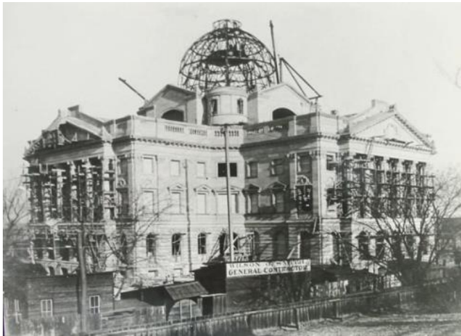
Luzerne County Courthouse circa 1908 River Street, under construction
