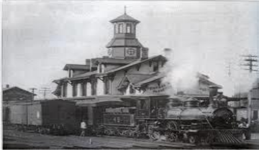
Functioning Central NJ Station in WB circa 1900
