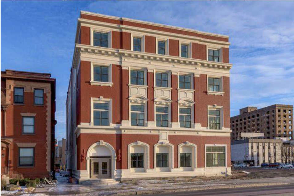
July 2022 – Sterling Annex Reborn with a new clean face-- Empty Sterling lot next door
